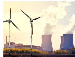
Nuclear power plant
